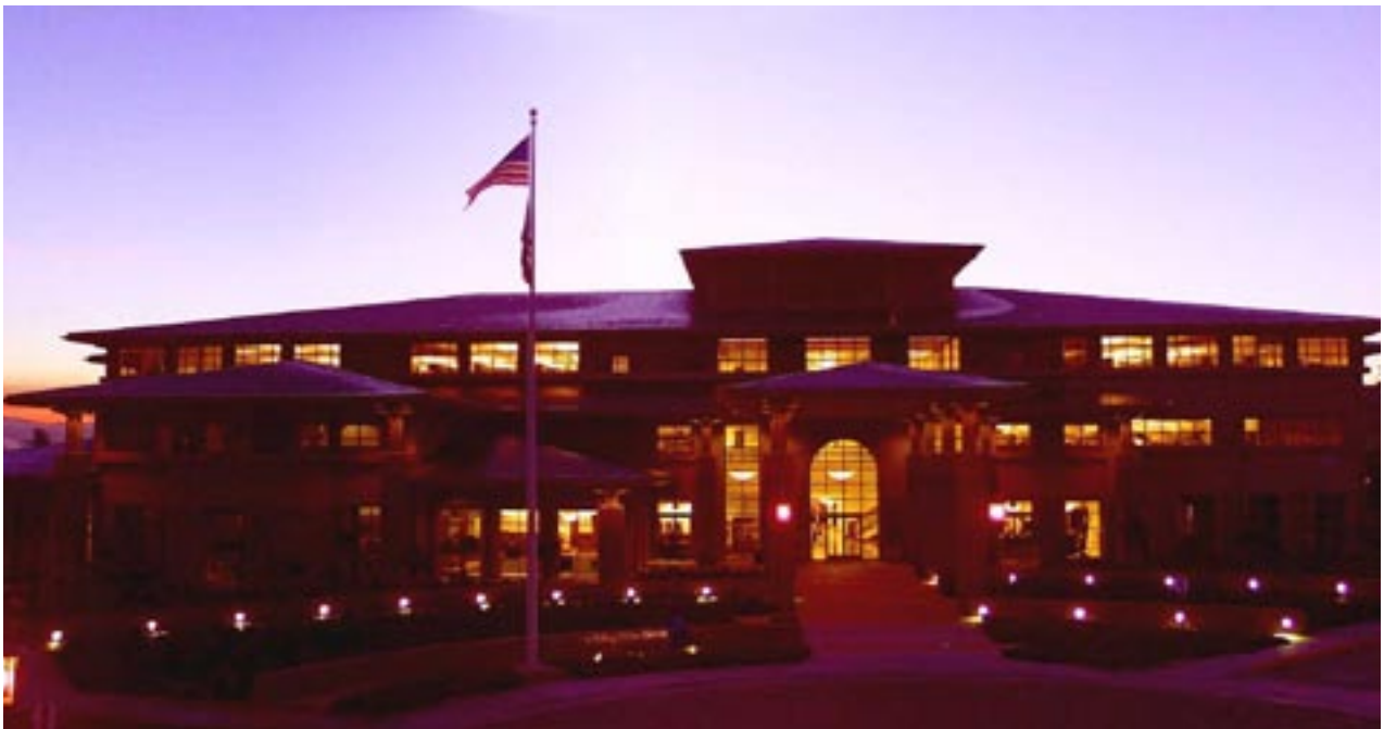
The District's solar panel arrays provide electricity for the headquarters campus.
